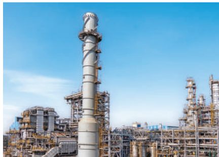
Ammonia Process Plant - Reformer Stack and Columns
