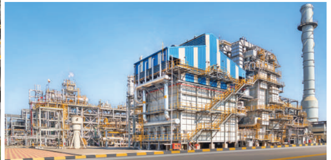
Ammonia Process Plant - Reformer Area
