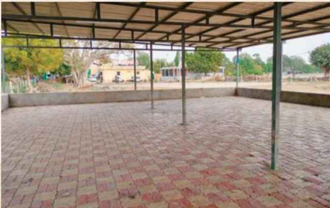
Construction of Shed and Paver Block at Dahej
