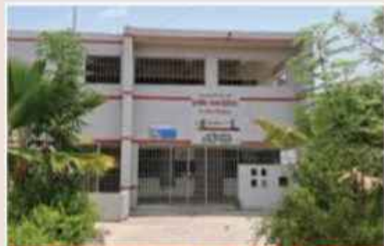
Classroom given a fresh look after renovation at Koliyad School, Dahej
