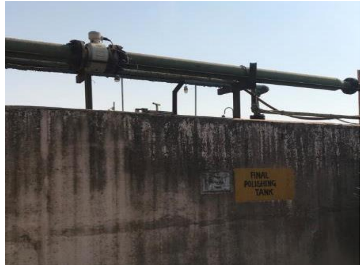
Flow meter at ETP-1 at K-1
