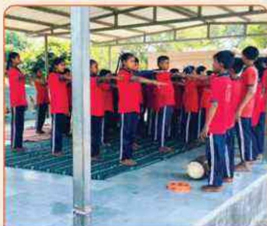
Flooring done at Koliyad primary school's mid-day meal area to improve facility and provide a better experience for students
