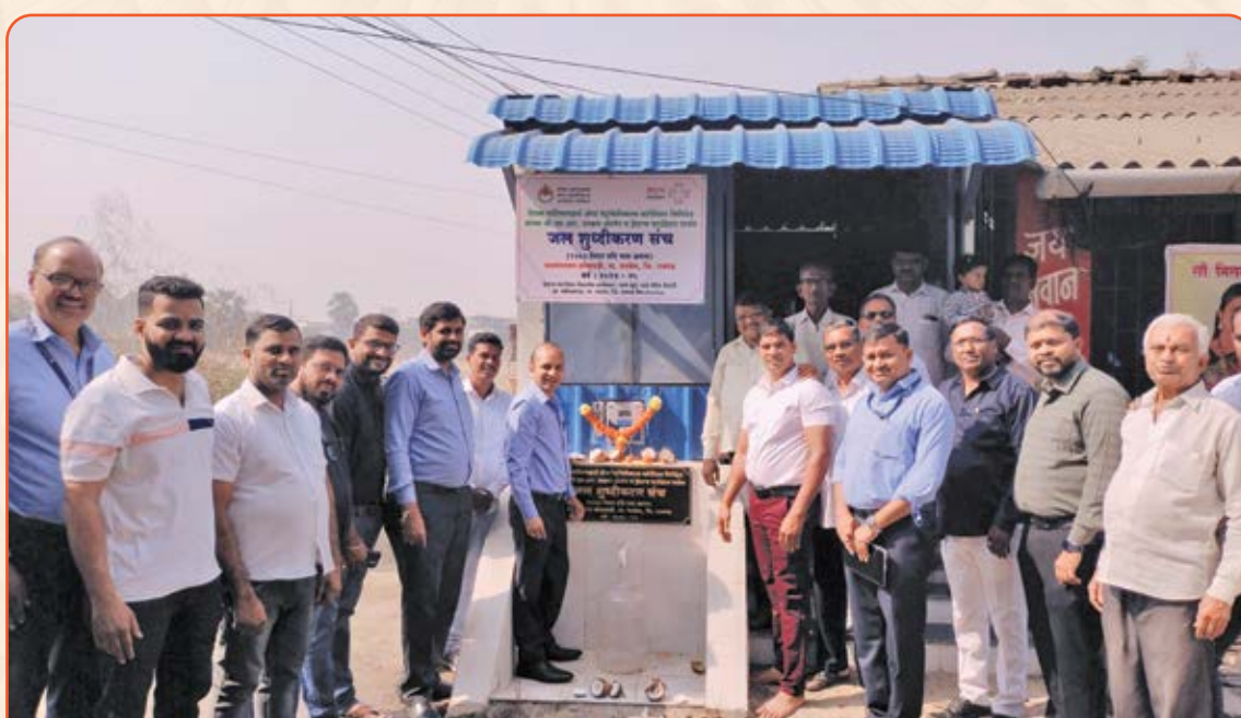
Installed community RO unit with water ATM in Kolwadi village to provide access to safe drinking water for all
