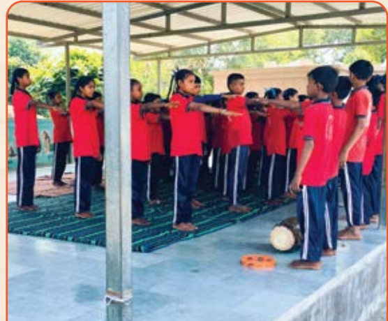
Flooring done at Koliyad primary school's mid-day meal area to improve facility and provide a better experience for students
